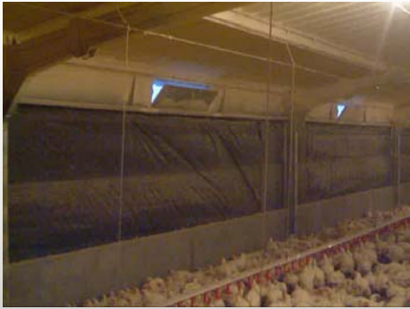
Air flow obstruction in open ceiling house
