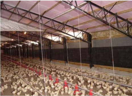
Open ceilings with exposed purlins, are a major obstruction
