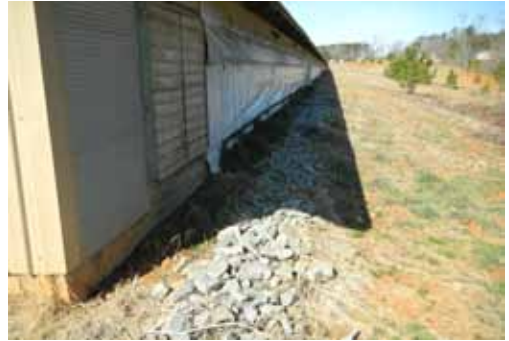
Figure 9. Rocks to prevent scouring
