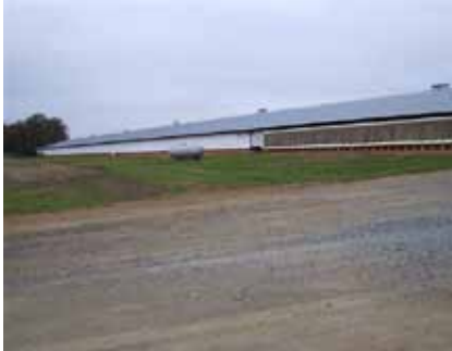
Figure 26. Poultry house with straight ridge line
