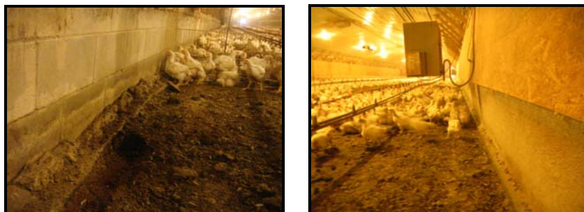
Figure 10. Soil should be added to maintain structural integrity
