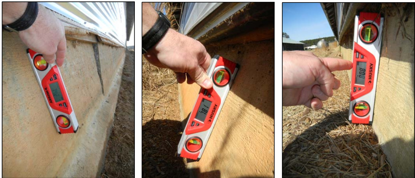
Figure 12. Measuring angle of rotation of concrete stem wall
