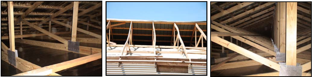
Figure 25. Bracing of trusses is essential to keep trusses vertical and to help carry loads along the length of house
