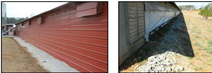
Figure 9. Rocks to prevent scouring
