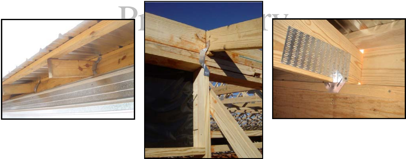
Figure 24. Trusses tied to top of wall using “hurricane straps”
