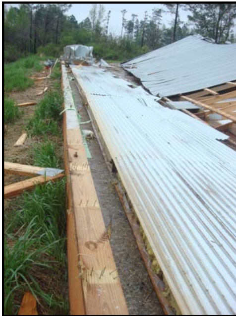
Figure 17. Nails loaded in withdrawal allowing pullout
