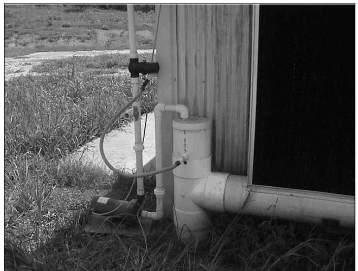
Figure 6. Centrifugal Pump
