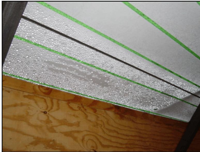
Figure 7. Condensation due to missing ceiling insulation
