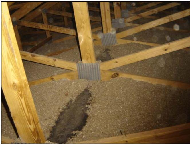
Figure 1. Missing blown ceiling insulation.
