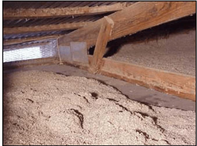
Figure 2. Missing ceiling insulation near side wall
