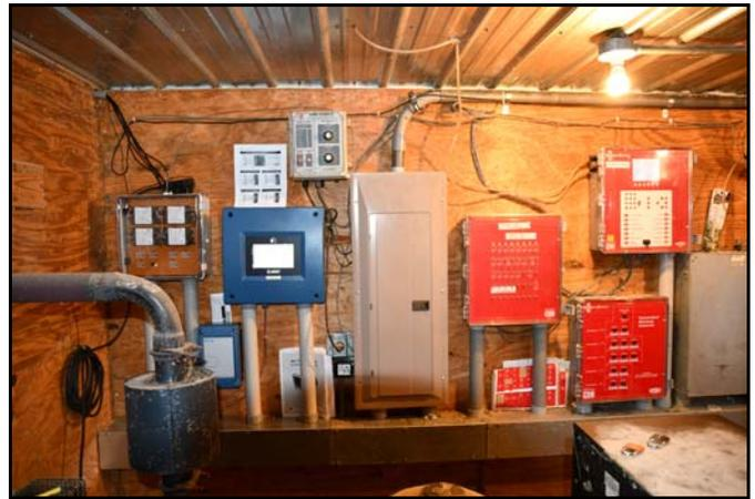
Figure 6. Choretime controller with Skov fan interface (blue box) and power meters (left)
