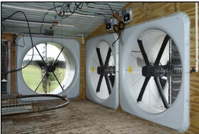
Figure 5. Variable speed 55" fans equipped with speed controllers (above fans).
