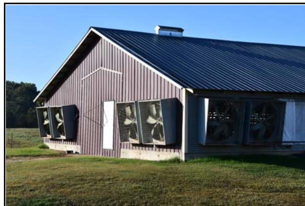
Figure 2. Traditional 1990's 48" slant-wall fan.
