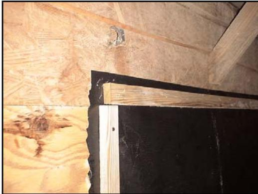
Figure 3. 1" X 2" wood strips securing Therm-All to side wall.
