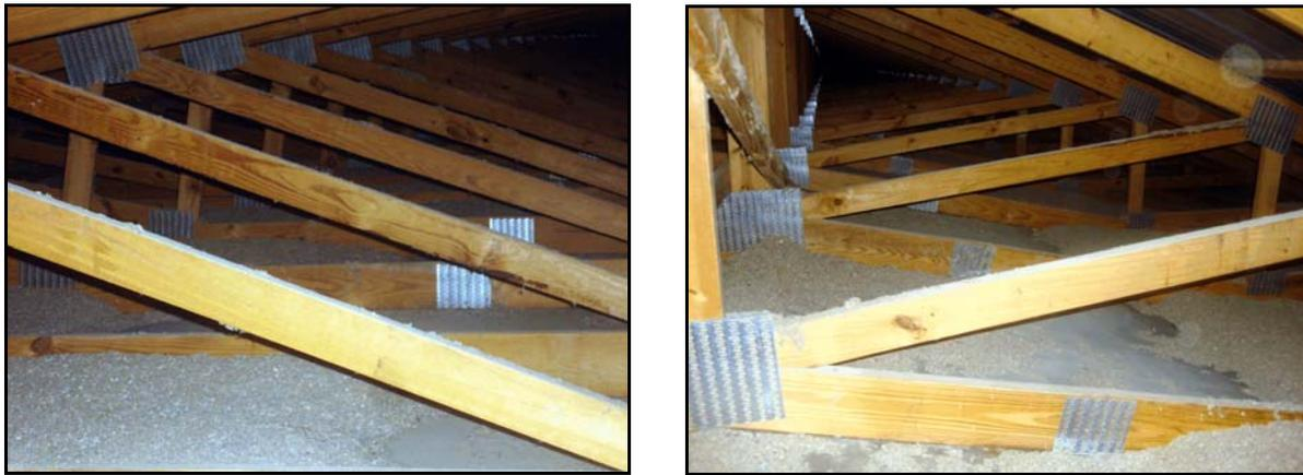
Figure 2. Missing ceiling insulation.
