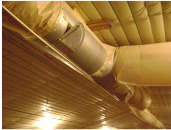
Figure 6. T-duct butterfly valve to aid in controlling hot air distribution
