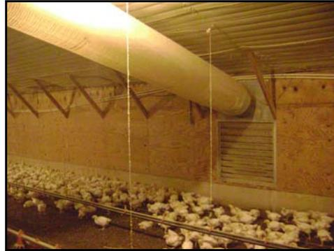
Figure 3. Heating unit air intake and flexible duct delivering hot air to T-duct
