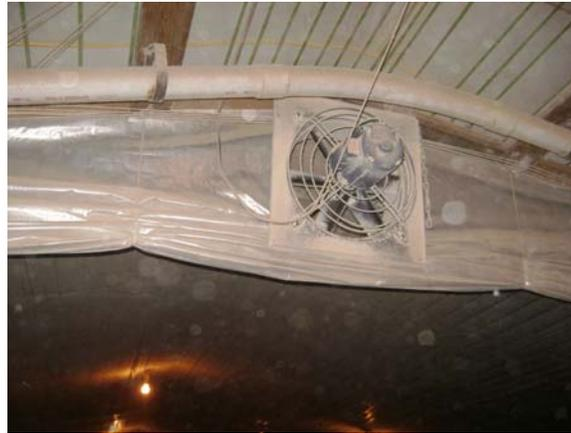
Figure 7. Circulation fan located in brooding curtain to deliver hot air to the nonbrooding end of the house
