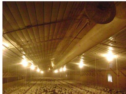
Figure 4. T-duct and perforated duct heat delivery system
