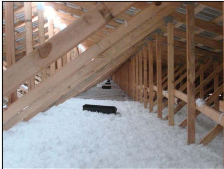
Figure 1. Blown stabilized fiberglass (foreground) and blown cellulose insulation (background)
