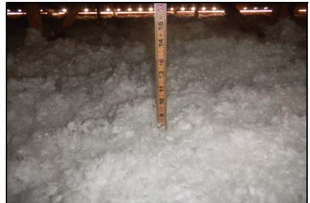
Figure 5. Blown stabilized fiberglass insulation (February, 2011. Two years and four months after installation)
