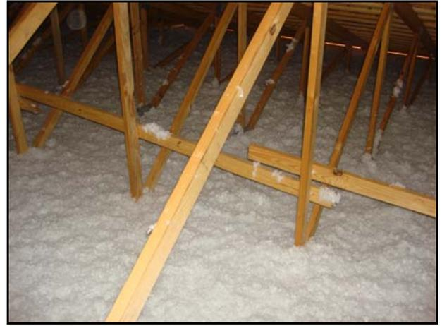
Figure 4. Blown stabilized fiberglass insulation (January, 2009. Three months after installation)
