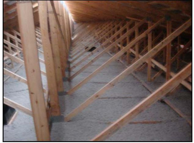
Figure 2. Blown cellulose insulation (January, 2009. Six months after installation)
