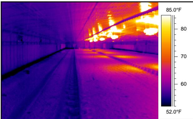
Figure 13. Quadratherms® installed down the center of a 50' wide house.
