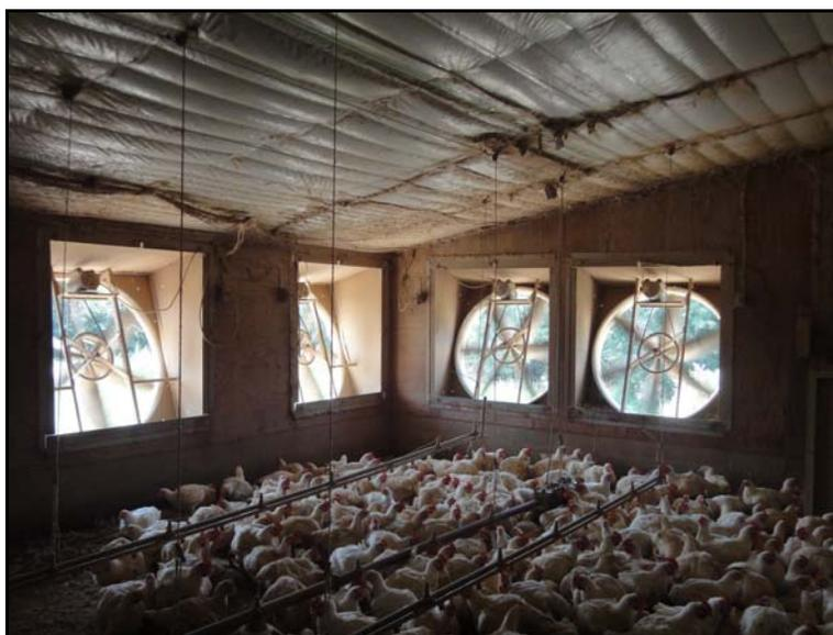
Figure 1. Adjacent tunnel fans operating in the corner of a tunnel-ventilated broiler house.
