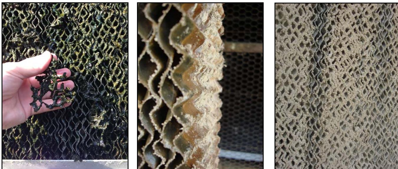
Figure 5. The static pressure required to pull air through a pad can increase dramatically when it is not regularly cleaned
