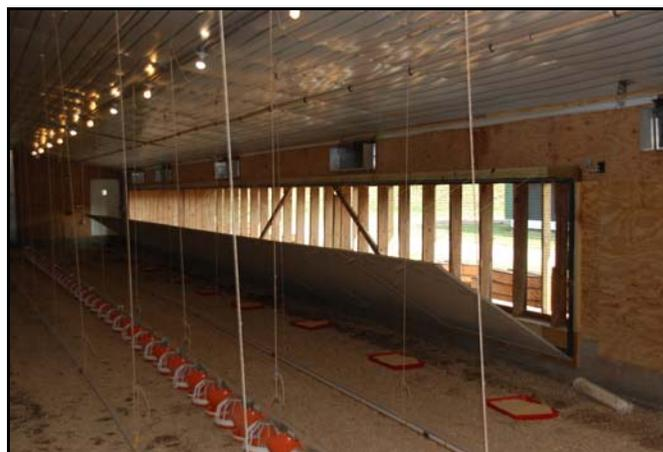
Figure 1. Study house with evaporative cooling pads removed.
