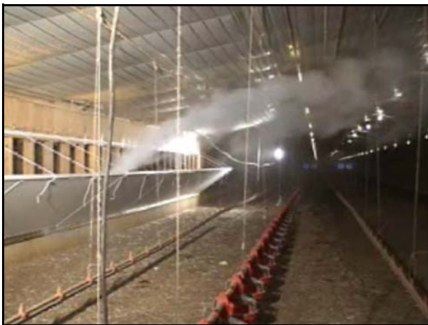
Figure 9. Air entering through tunnel doors moving along the ceiling then back toward the side wall at floor level.
