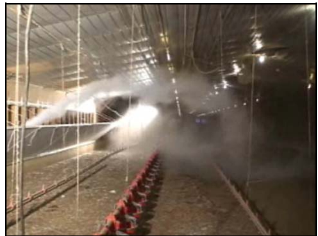
Figure 9. Air entering through tunnel doors moving along the ceiling then back toward the side wall at floor level.
