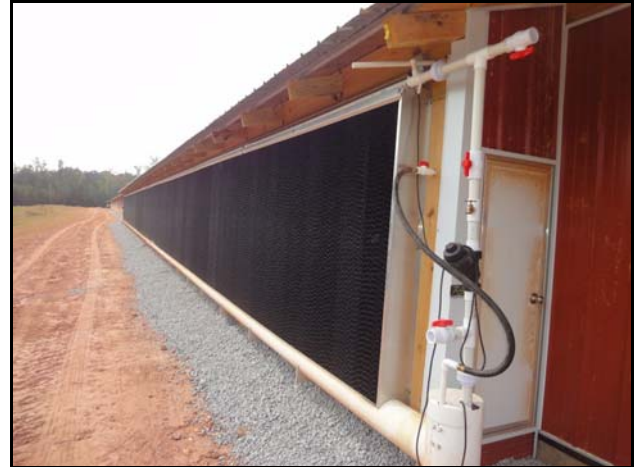
Figure 2. Six-foot-tall pad system.
