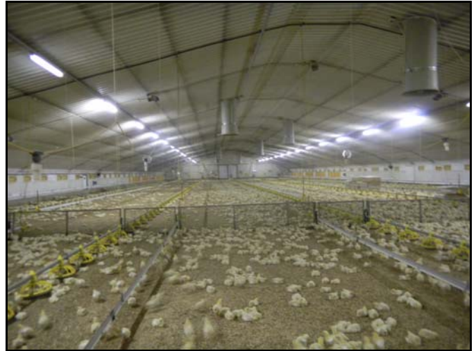
Figure 6. High ceiling in a relatively cold climate.
