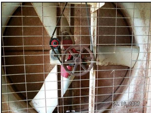
Figure 11. Rust on fan with butterfly shutters
