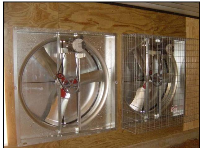
Figure 6. Interior view of butterfly shutter fan
