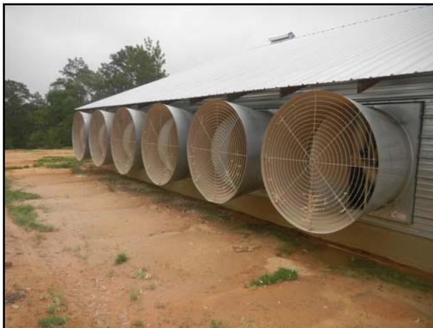
Figure 5. Tunnel fan with butterfly shutters
