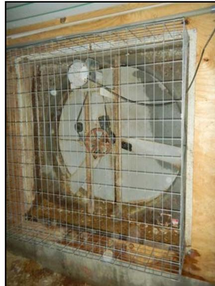
Figure 10. Condensation formation on fan surfaces and components
