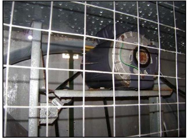
Figure 8. Condensation forming on fan surface
