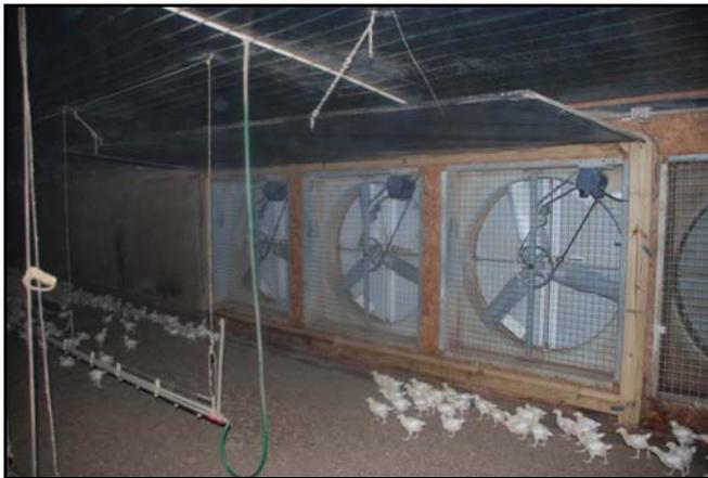
Figure 11. Butterfly shutter fans with cover
