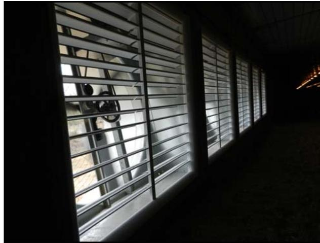
Figure 3. Interior shutters of fan with slant wall housing
