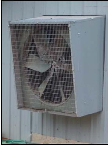
Figure 2. Slant wall housing
