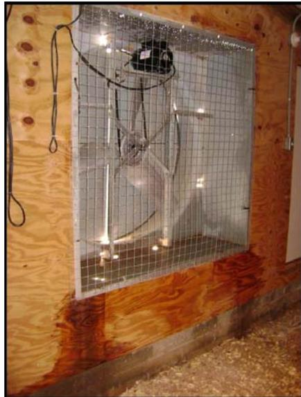
Figure 9. Condensation formation on fan surfaces and components
