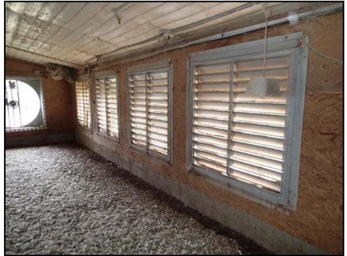
Figure 5. High static pressure, 48" fans shutters partially closed.
