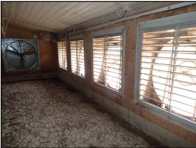
Figure 4. Low static pressure, 48" fans shutters fully opened.
