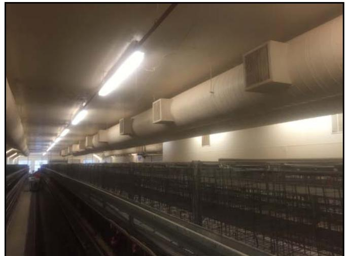
Figure 5. Positive pressure duct system
