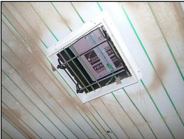
Figure 10. View of butterfly shutter with lower portion of attic inlet removed (fan off).
