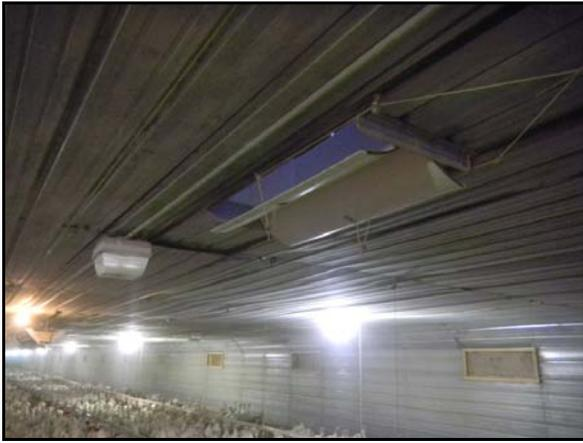
Figure 24. Excessive attic inlet opening.
