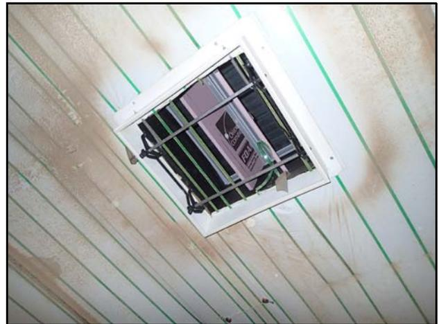
Figure 11. View of butterfly shutter with lower portion of attic inlet removed (fan on).
