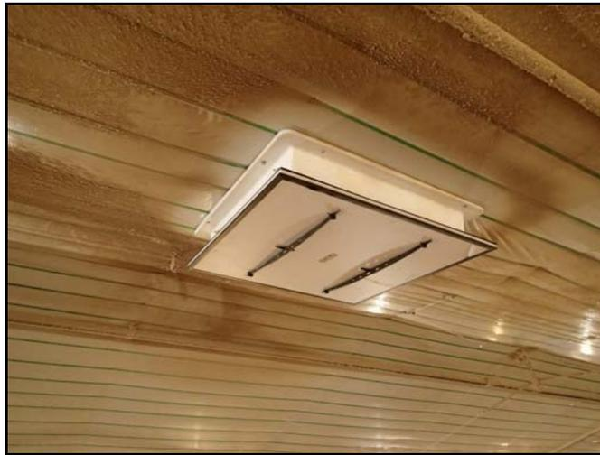
Figure 9. Counter-weighted attic inlet.
