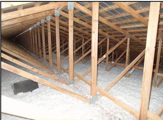
Figure 6. Blown stabilized fiberglass (7 years)
