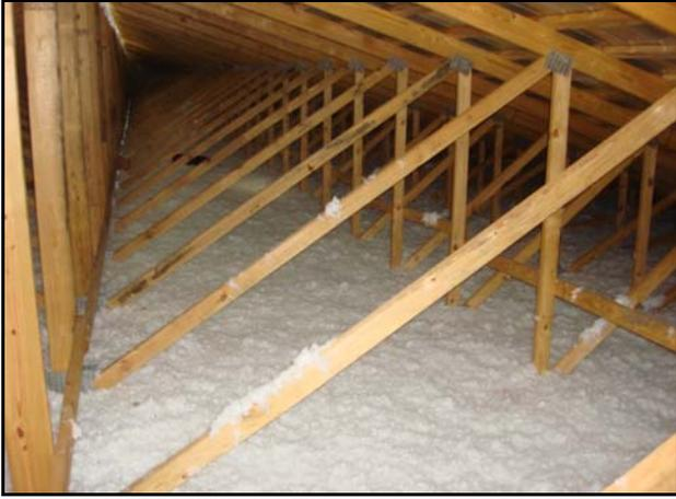
Figure 2. Blown stabilized fiberglass (6 months)
