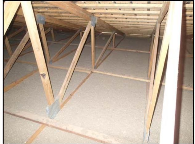
Figure 9. Blown cellulose insulation (7 years)
