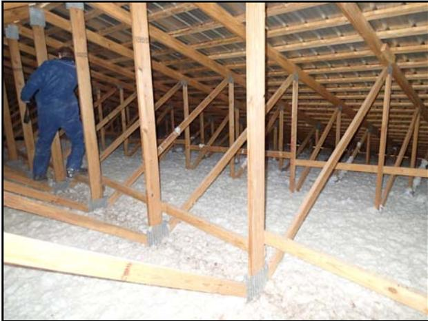
Figure 8. Blown stabilized insulation (7 years)
