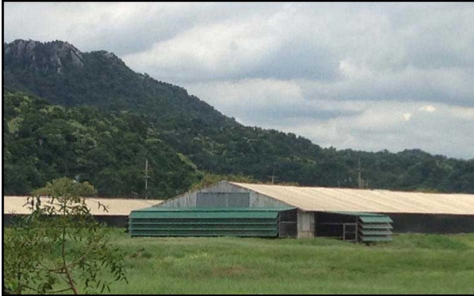
Figure 13. Shades installed on tunnel fans to reduce the amount of light entering the house through operating tunnel fans.
