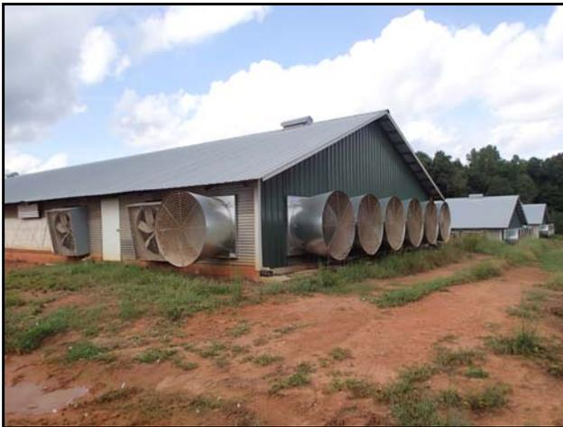
Figure 3. Tunnel fans in end wall
