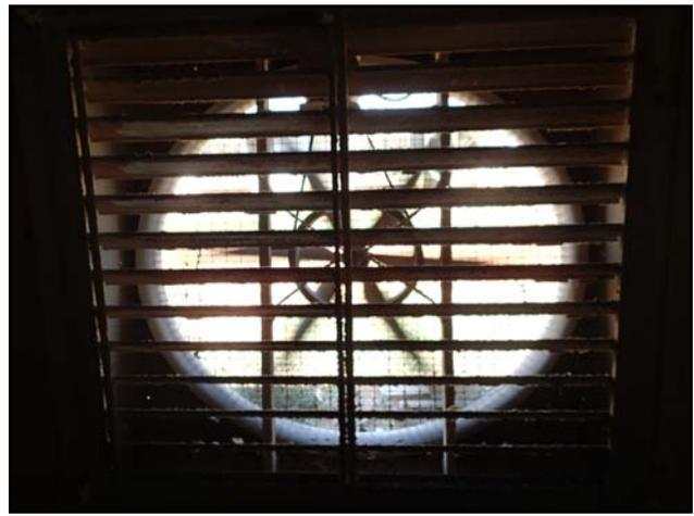
Figure 2. Light entering through tunnel fan with traditional interior shutter.
