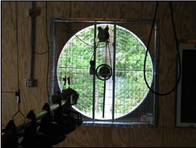
Figure 1. Light entering through tunnel fan with butterfly shutter.
