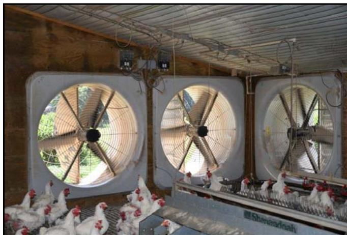
Figure 2. 55" Variable-speed tunnel fans (interior view).
