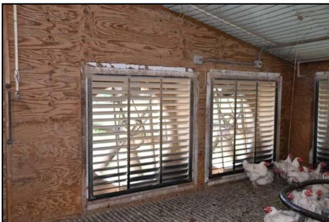
Figure 3. 48" fans at end of breeder flock.
