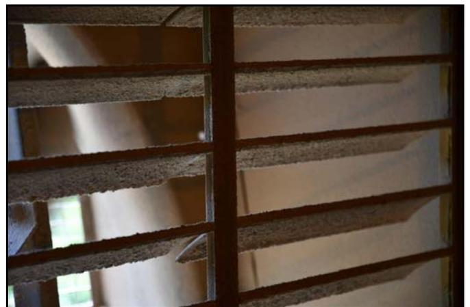
Figure 4. Dust accumulation on fan shutters.
