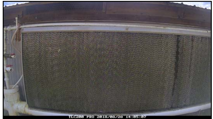
Figure 3. Evaporative cooling pad at 2:05 pm - Day 1 (temperature and interval timer)
