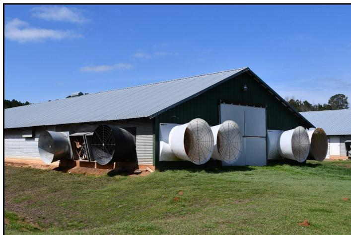
Figure 2. Retrofitted house where four of the 48" fans were replaced with four variable-speed 54" fans.
