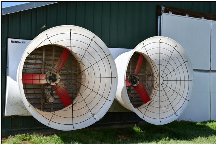
Figure 3. Variable-speed Multifan 54" Tunnel Fan.
