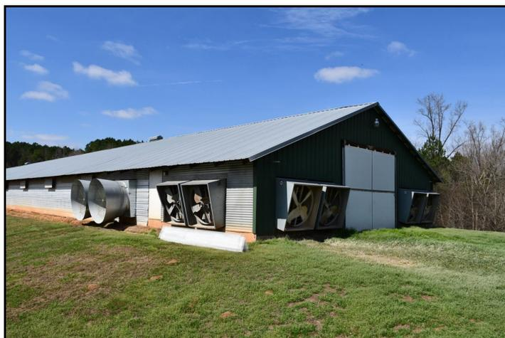
Figure 1. Tunnel-ventilated house equipped with eight 48" fans and four 54" cone fans.
