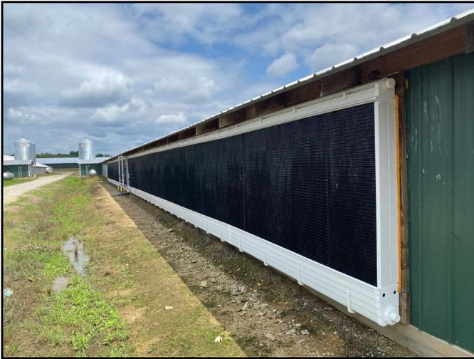
Figure 1. New plastic pads - new system
