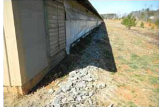
Figure 9. Rocks to prevent scouring
