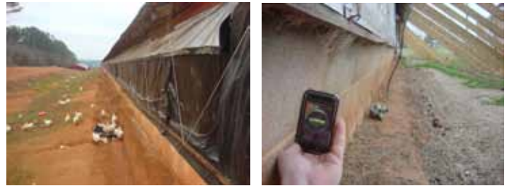
Figure 13. Rotation of concrete block wall foundation
