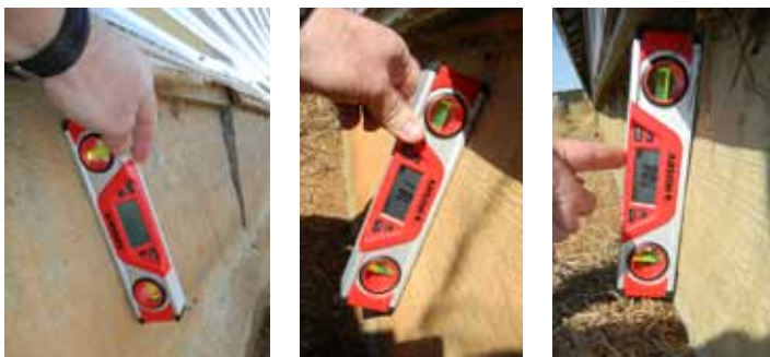
Figure 12. Measuring the angle of rotation of a concrete stem wall
