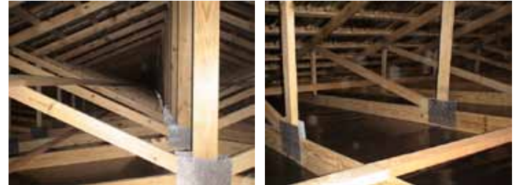
Figure 25. Bracing of trusses is essential to keep trusses vertical and to help carry loads along the length of the house
