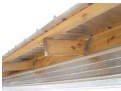
Figure 24. Trusses tied to the top of a wall using "hurricane straps"
