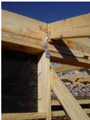
Figure 24. Trusses tied to the top of a wall using "hurricane straps"
