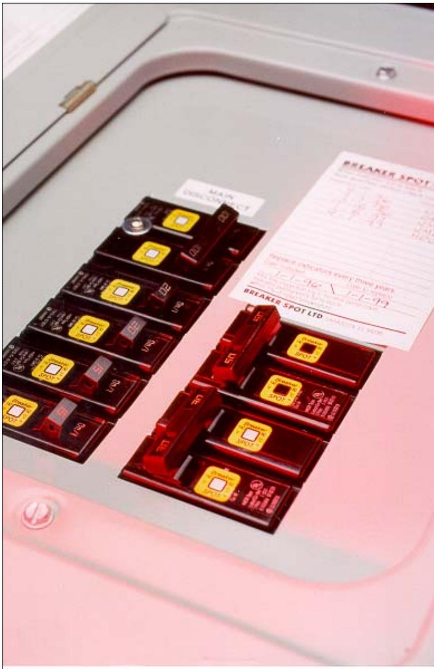
Figure 2. Temperature indicators should be installed on each line of a 240 volt circuit breaker. The temperature indicators on the top, right circuit breaker have turned black, indicating a high temperature condition has occurred.
