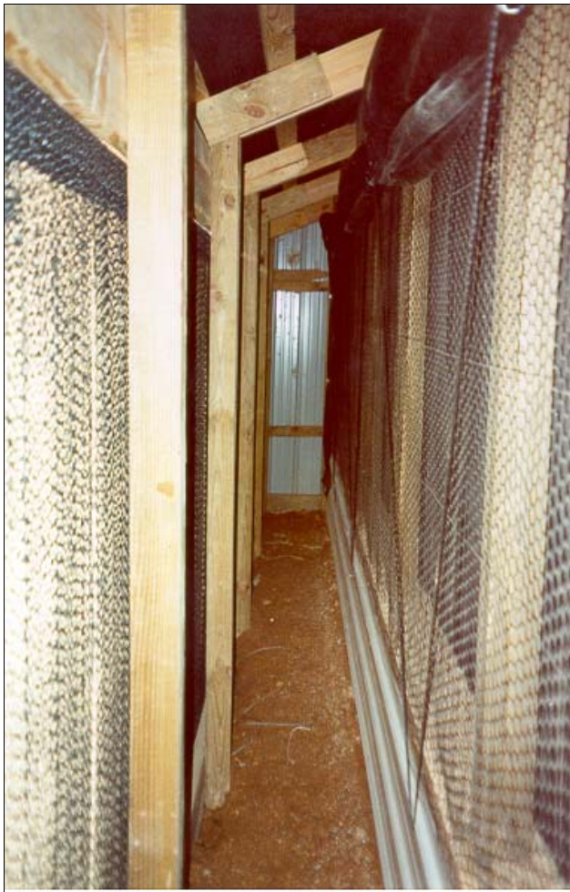
Figure 2. Evaporative cooling pad structure
