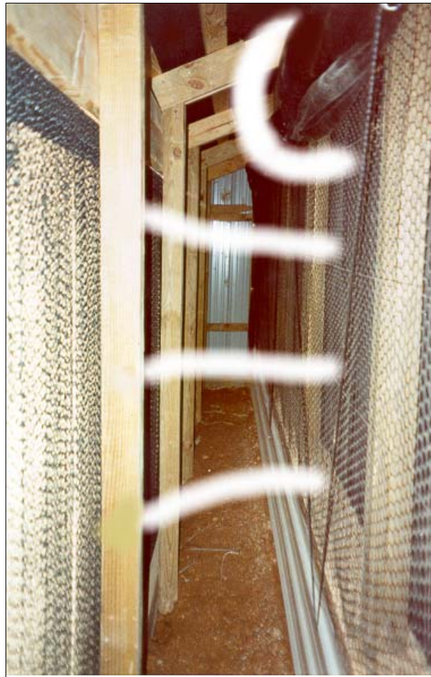
Figure 3. Illustration of air being pulled through an evaporative cooling pad as well as from the attic space by tunnel ventilation fans.
