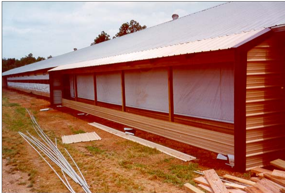
Figure 1. Evaporative Cooling Pad Structure - Without Pads
