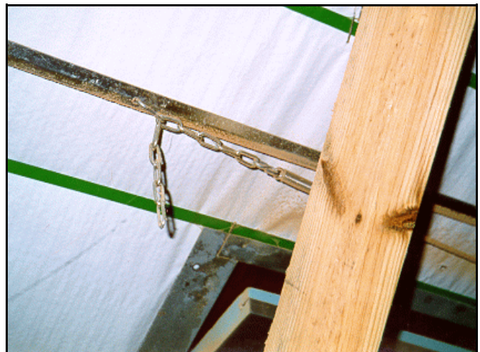
Figure 2. Inlet attached to steel banding strip
