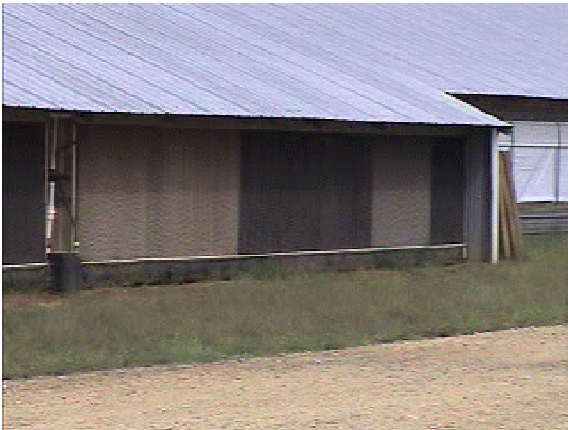
Figure 1. Different types of pads. The light pads on the left are the StayCool® (far left) and Glacier-Cor® (left) with surface coating. The dark pads in the center are Kuul® (left center) and Munters® pads (right center) with surface coating. The gray section, toward the right, between the two black sections is the black Kuul® pad and the section of black pad at the far right is again the surface coated Munters® pad.
