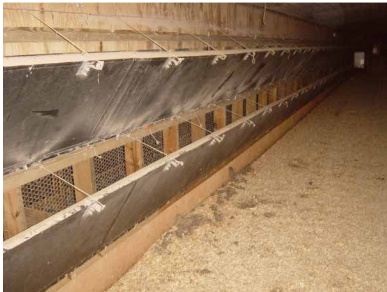
Figure 3. Partially Opened Tunnel Doors
