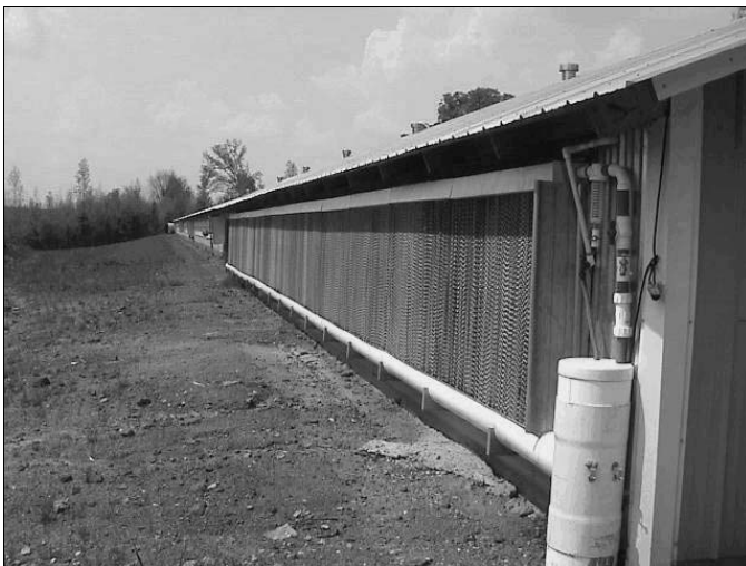
Figure 7. 70' system with pump on end
