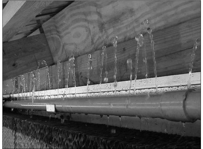
Figure 5. Water column height (near pump 70' system) Figure 6. Water column height (far end of same system)
