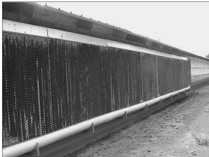
Figure 3. Proper water flow
