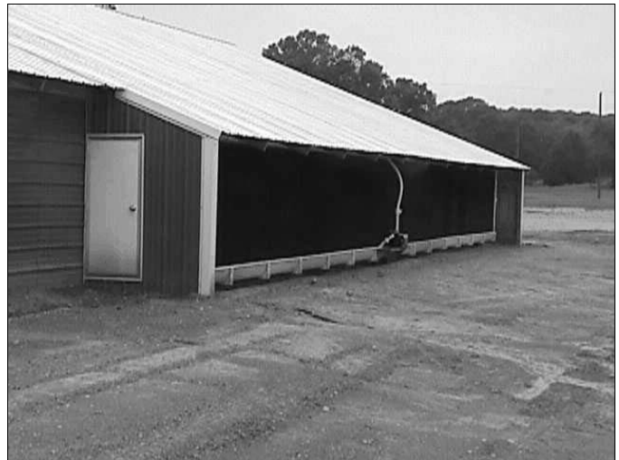
Figure 8. 60' system with pump in center
