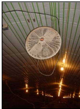
Figure 1. 1/15 h.p. circulation fan
