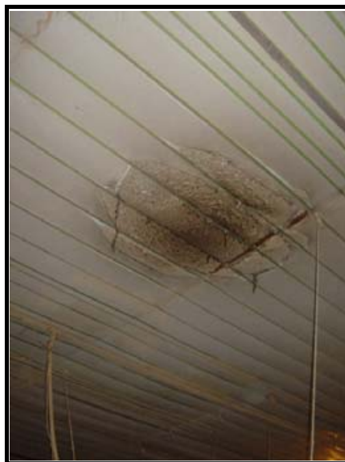
Figure 2. Ceiling fire damage
