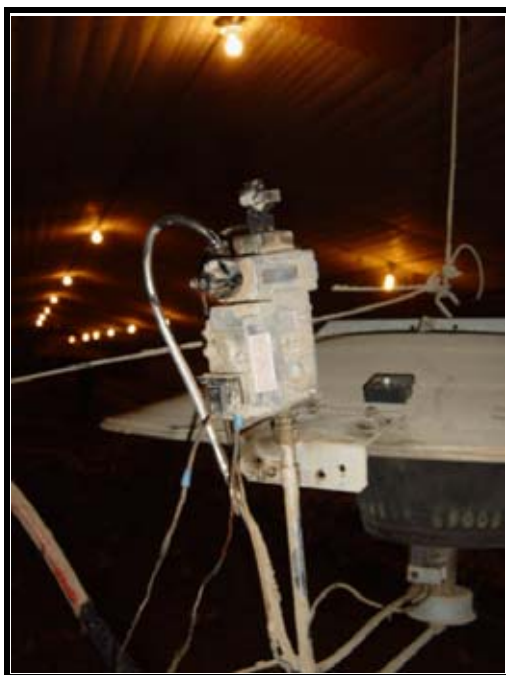
Figure 1. Fire caused by gas leakage where hose attaches to brooder
