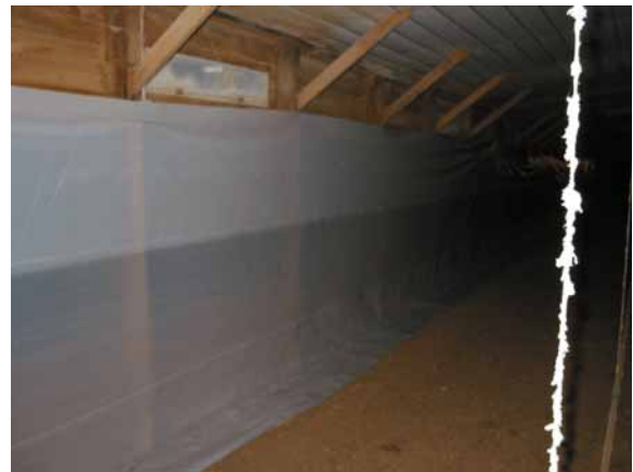
Figure 9. 4" X 6" post side wall with plastic sheeting.
