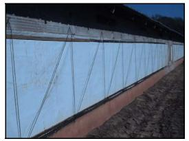
Figure 4. Side wall curtain sealed using 1" X 2" wood strips.
