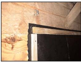
Figure 3. 1" X 2" wood strips securing Therm-All to side wall.
