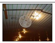
Over the last couple of years 1/15 hp circulation fans have been installed on hundreds of farms across the U.S. The vast majority of producers have found the fans to reduce fuel usage, keep house temperatures more uniform, and improve litter conditions. As with any new product, a number of lessons have been learned as to how to get the most out of 1/15 hp circulation fans. The following are a few points to consider when installing and operating 1/15 hp circulation fans:
