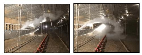
Figure 4. Air entering through tunnel doors.
