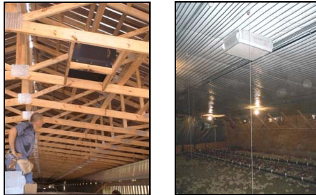
Figure 1. Framing for attic inlet with insulation guard installed.
