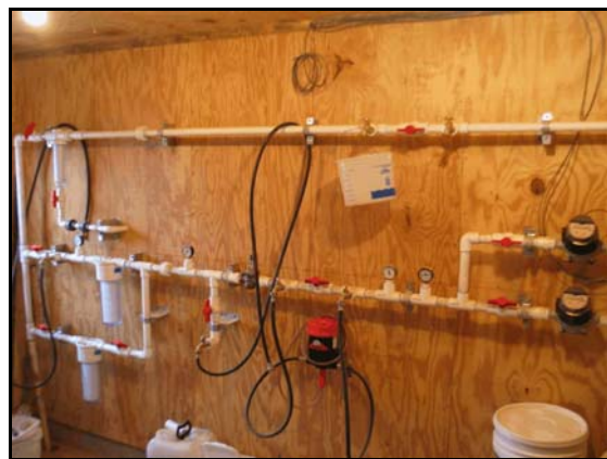
Figure 2. Water panel with two water meters.
