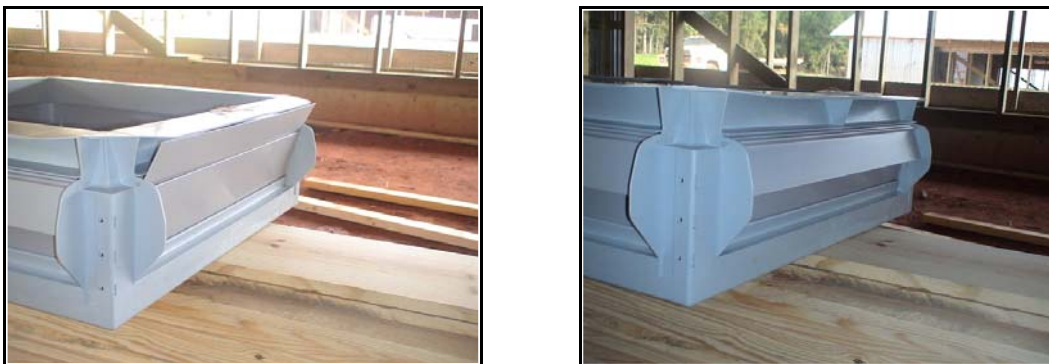
Figure 5. Attic inlet with top blade in open and closed/locked positions.
