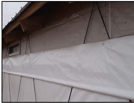
Figure 4. Poorly installed curtain pocket and a thermal image of the same side wall on a cold morning.
