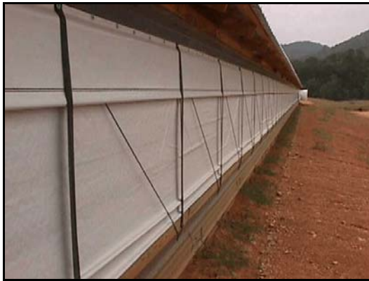
Figure 3. Properly installed curtain pockets with the bottom of the curtain stripped with wood.
