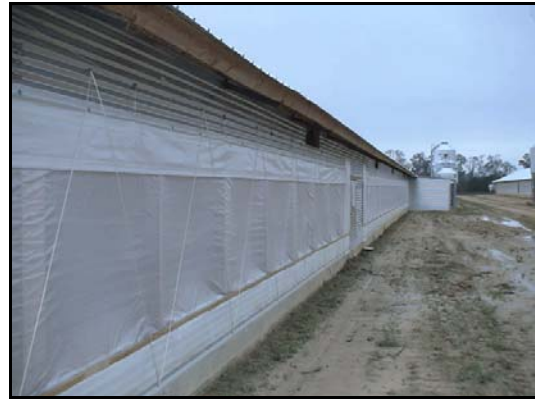
Figure 3. Properly installed curtain pockets with the bottom of the curtain stripped with wood.
