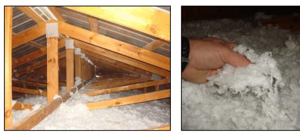
Figure 1. Blown stabilized fiberglass insulation.
