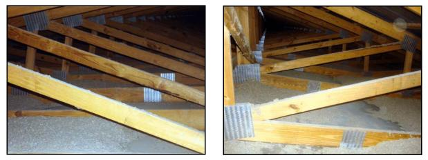
Figure 2. Missing ceiling insulation.
