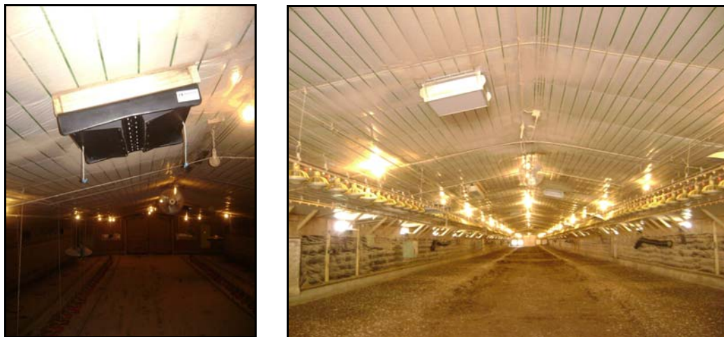
Figure 4. Two way and four way attic inlets introducing fresh air in the center of the house.
