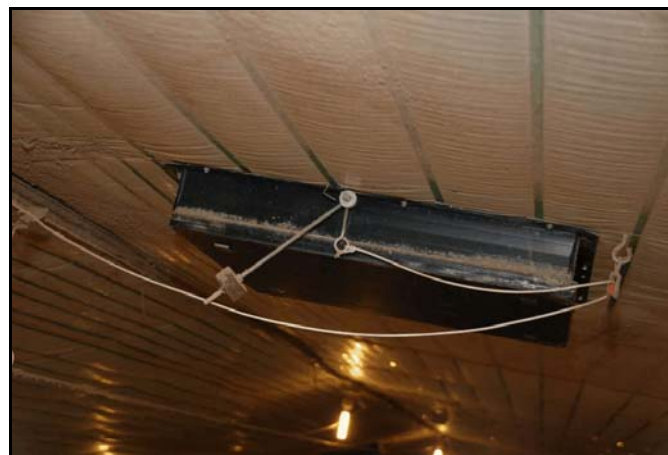
Figure 5. Attic inlet's counterweight
