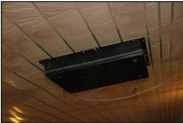
Figure 1. New attic inlet in closed position.
