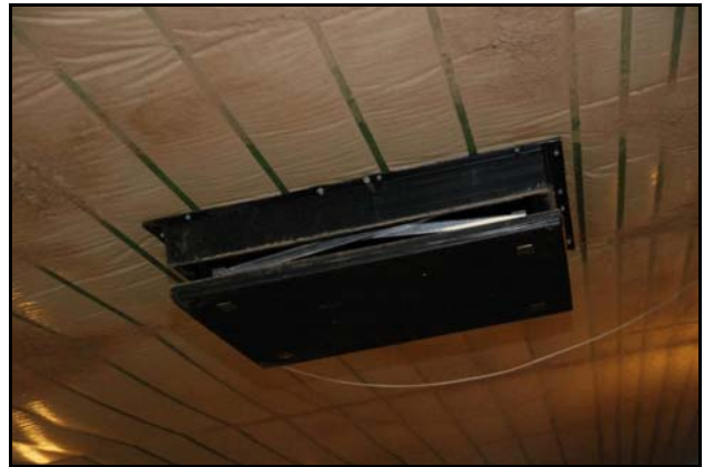
Figure 2. New attic inlet partially open.
