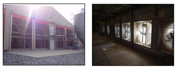
Figure 1. Tunnel-ventilated commercial layer house
