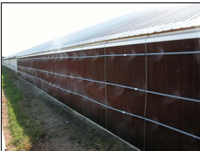
Figure 9. Two inch fogging-pad system
