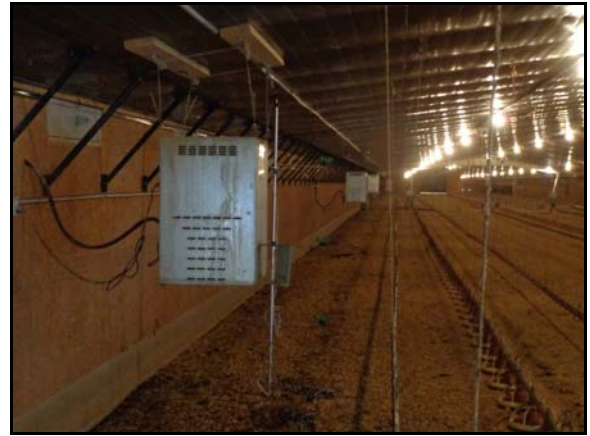
Figure 5. Furnaces four feet above floor.
