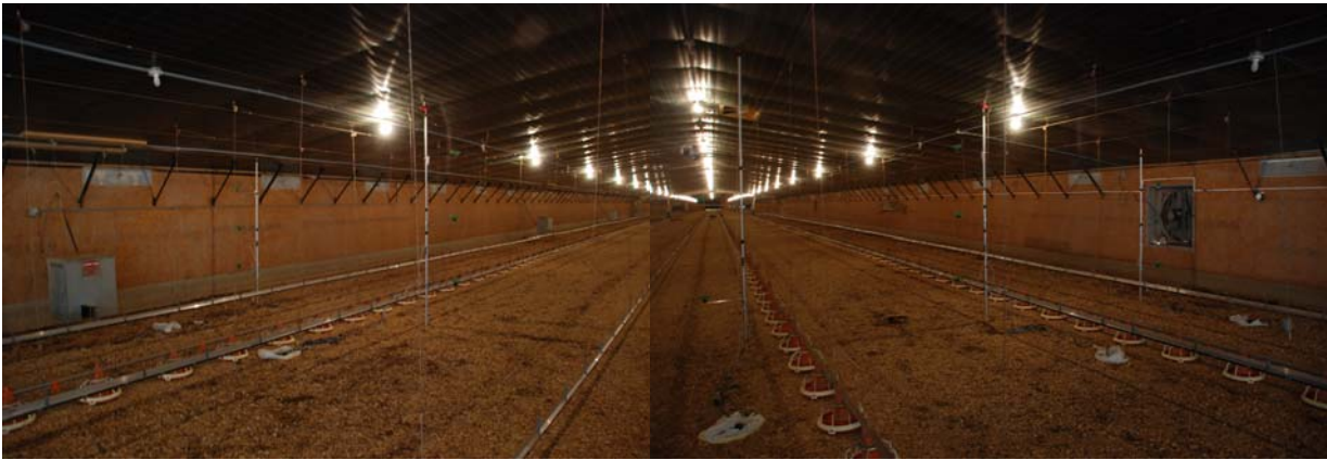
Figure 1. Air velocity poles in a 50' X 560' totally enclosed broiler house.
