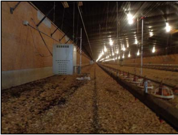
Figure 4. Furnaces one foot above floor.
