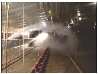
Figure 6. Air flow pattern in house equipped with tunnel inlet doors.
