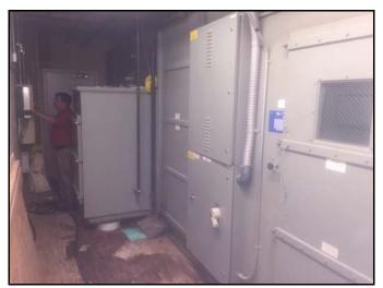
Figure 6. Positive pressure air handling system
